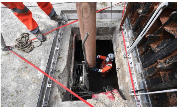
Agent Assainissement, intervention CATEC
